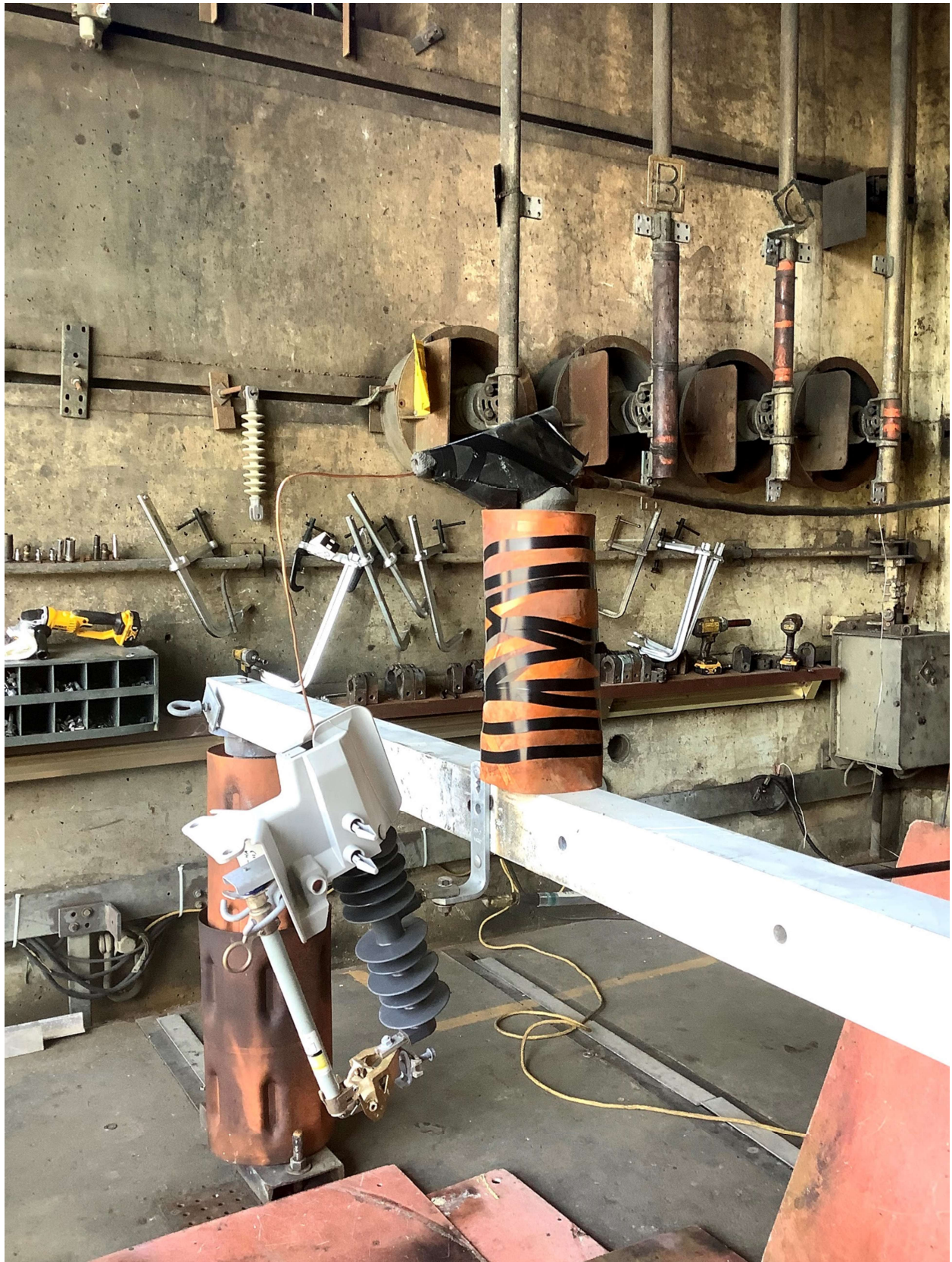
Figure 10. Setup for the high current (power arc) tests.
