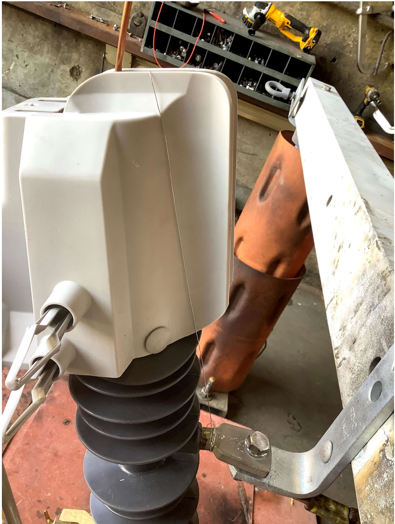
Figure 11. Setup for the high current (power arc) tests, fuse wire.
